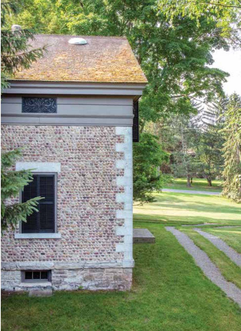
LEFT Cobblestone masonry is laid up with lime mortar. Dressed stone was used for window lintels and corner quoins.
